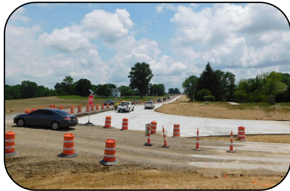
Refugee Road Widening Project
