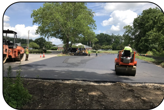
Victory Park - Parking Lot Expansion
