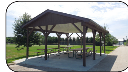
Diley Road Softball Fields Shelter 2
