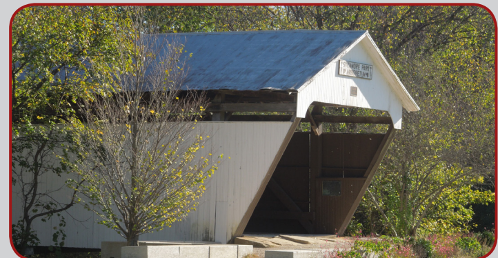
Covered Bridge at Sycamore Creek Park
